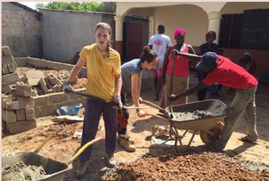
Darla and colleagues preparing concrete mix
