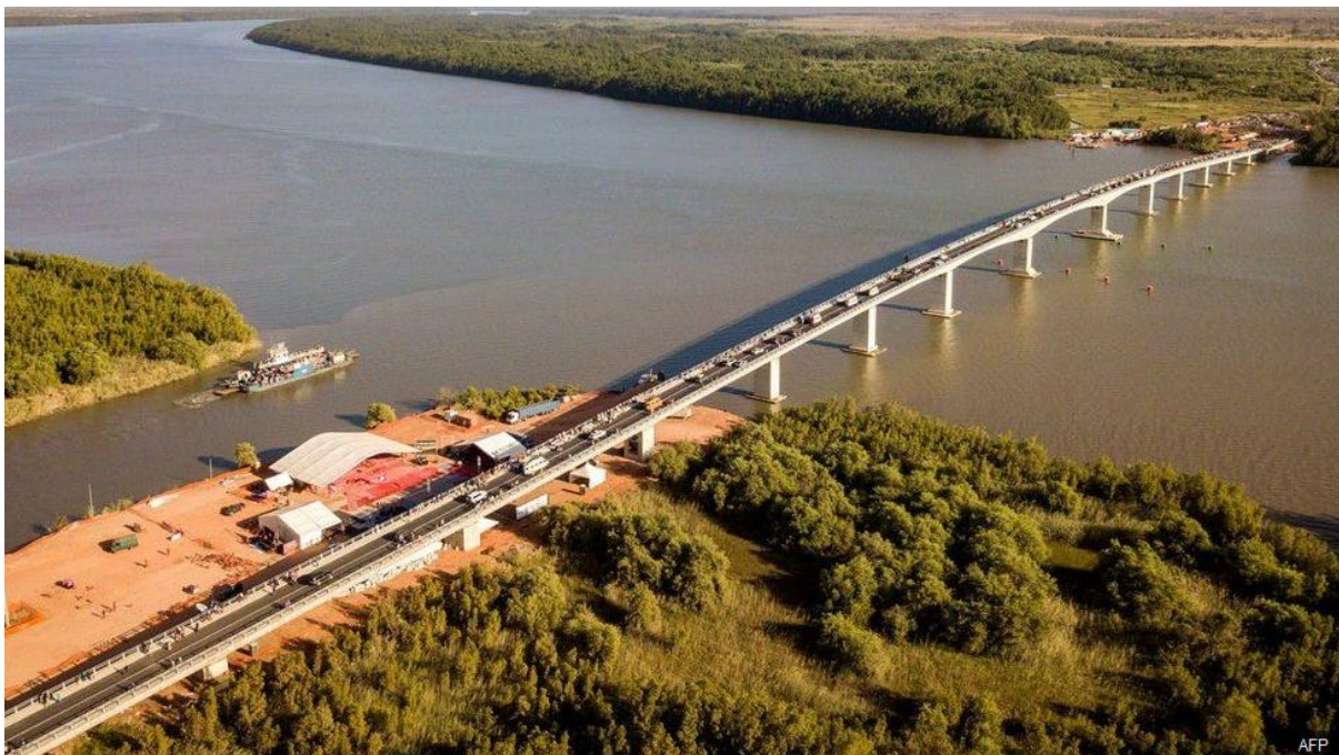
The new bridge over the River Gambia at Farafenni.
